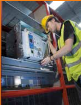
Direct Response Engineer Installing Retrofit ACB
